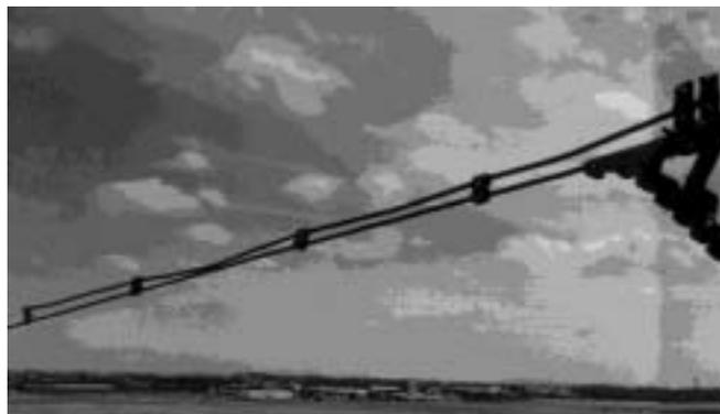
**Inverted BATE Damper at Strain Clamp**
