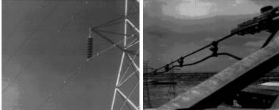
**Modified BATE Damper | BATE Damper at Strain Clamp**
